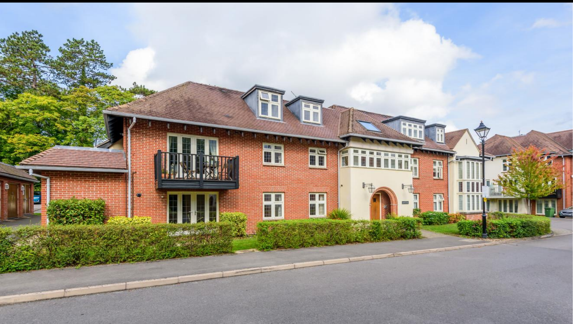
Queens Lodge, Highcroft Road, Winchester, Hampshire, SO22 5GT
