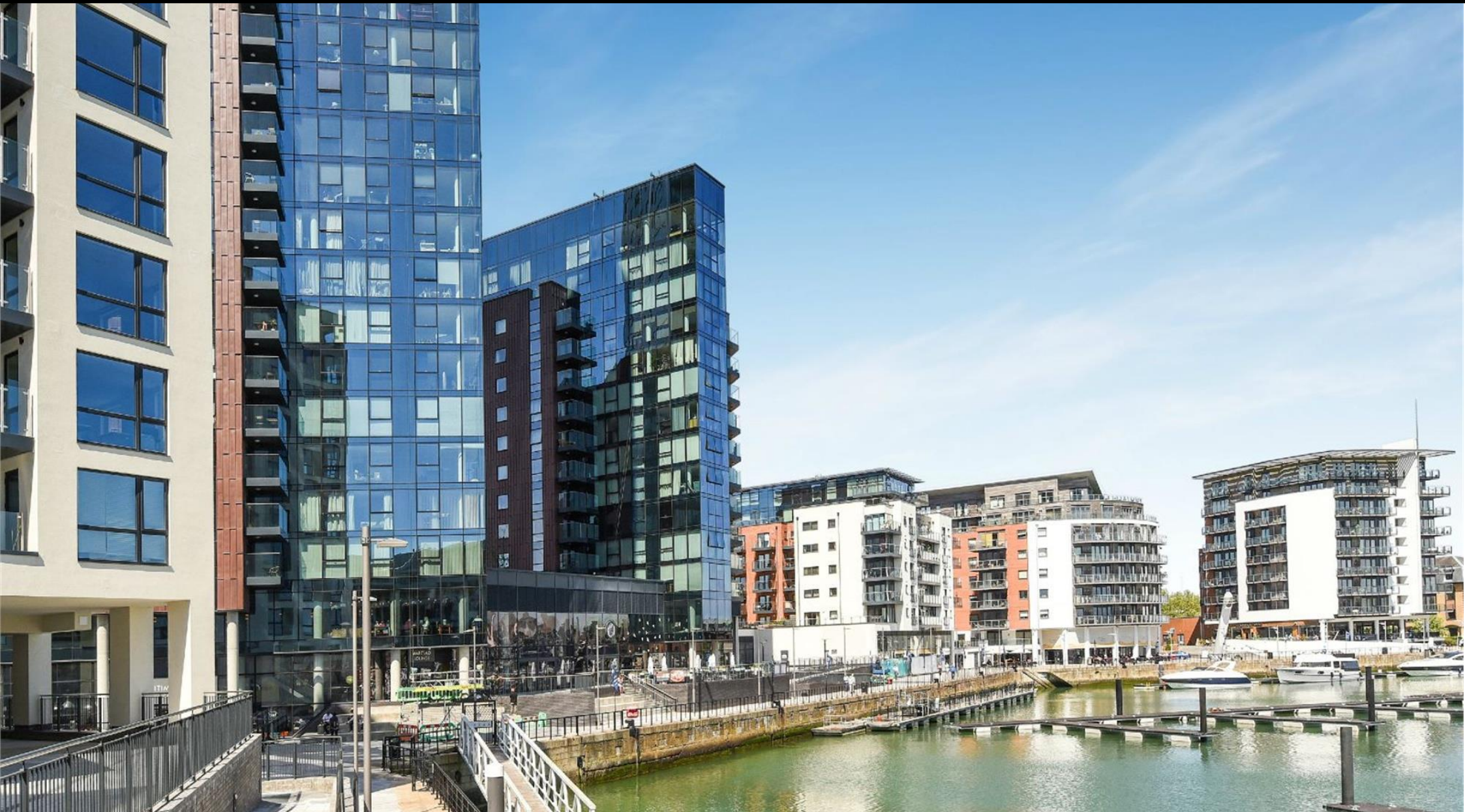
165 The Hawkins Tower, Admirals Quay, Ocean Way, Southampton, Hampshire, SO14 3LH
