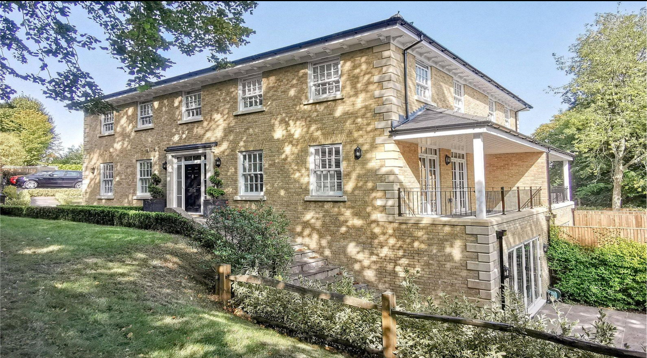
Chilbolton Gate, Chilbolton Avenue, Winchester, Hampshire, SO22 5HD
