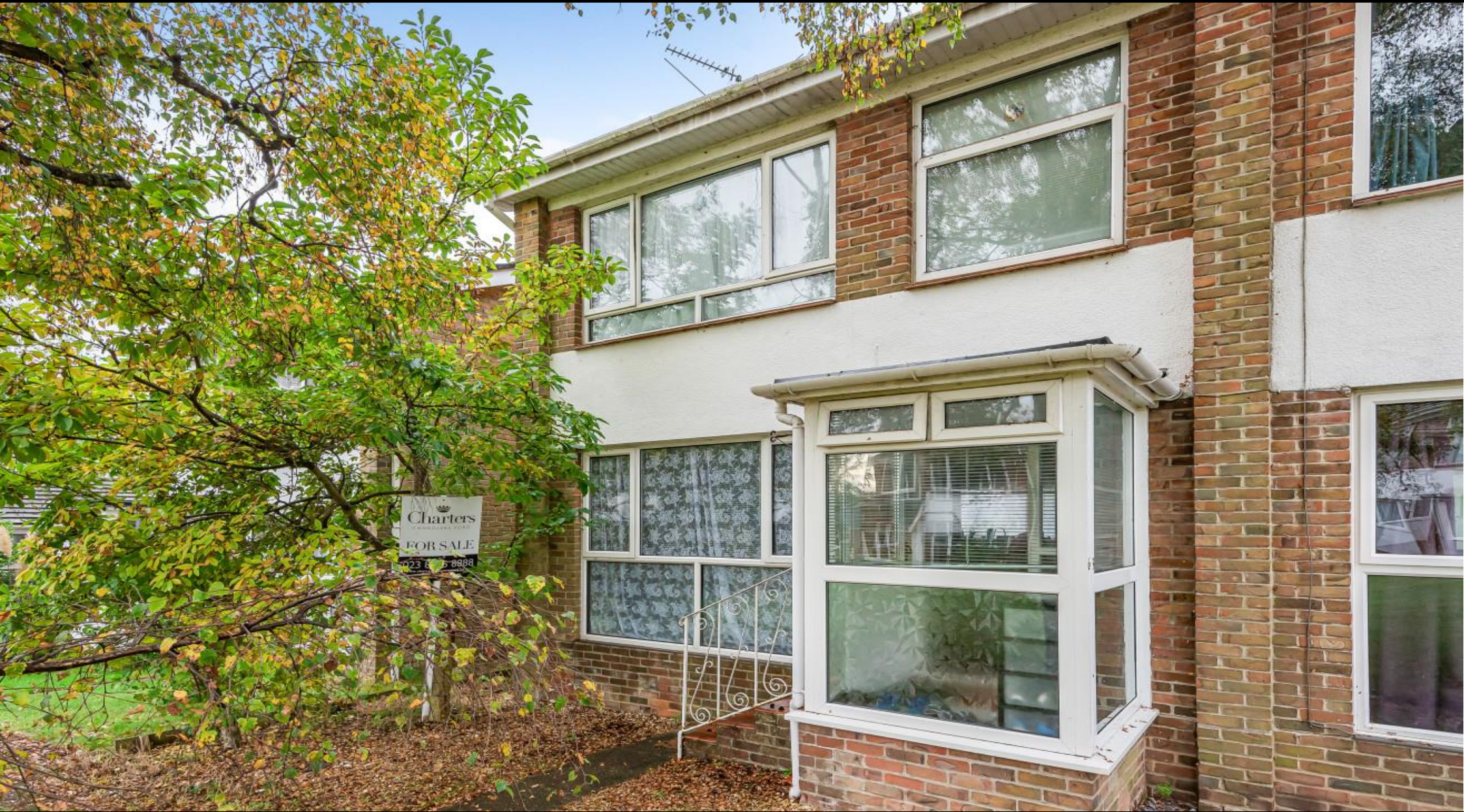
Sycamore Avenue, Chandler's Ford, Hampshire, SO53 5RG
