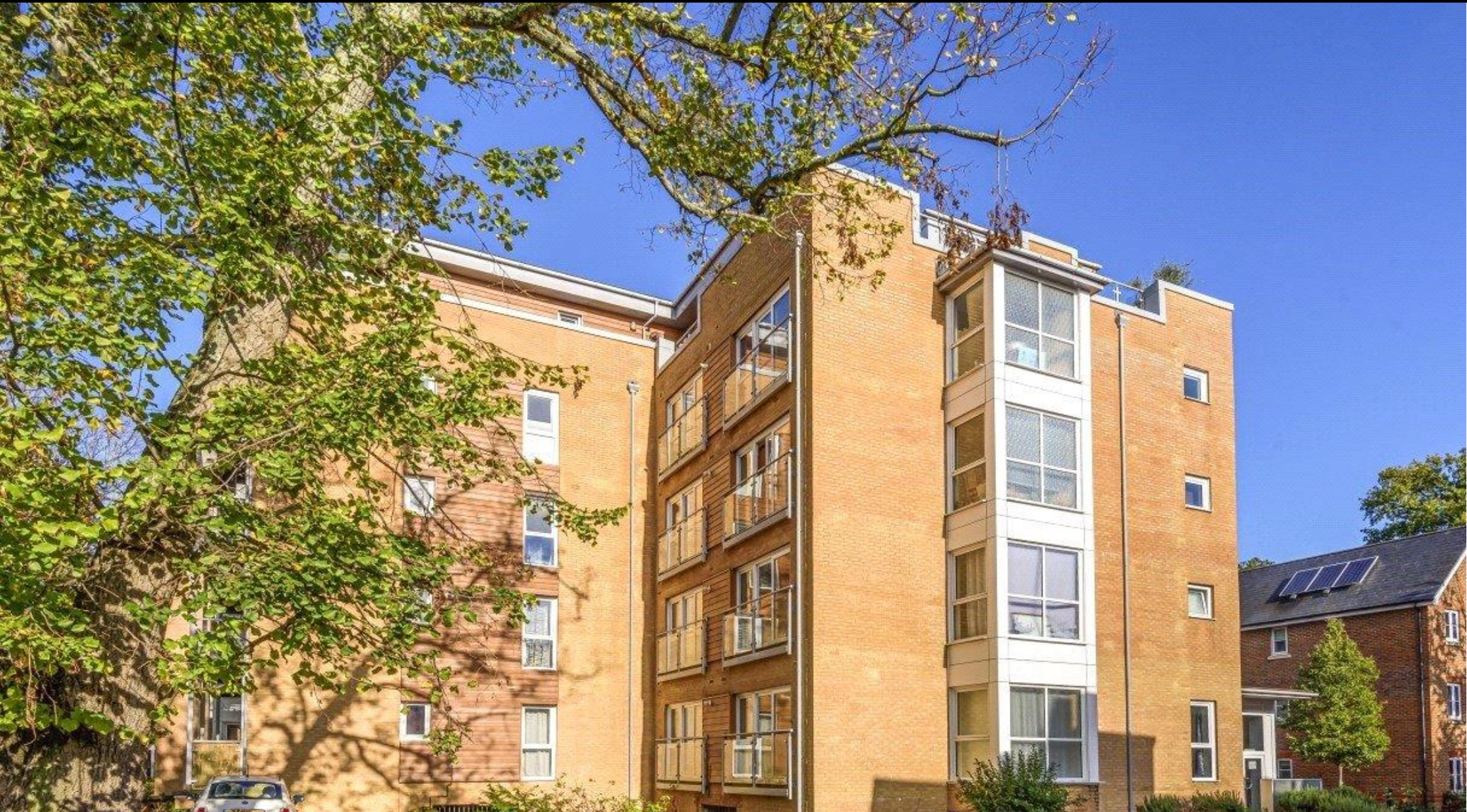
Alexander Place, 87 The Avenue, Southampton, Hampshire, SO17 1YB
