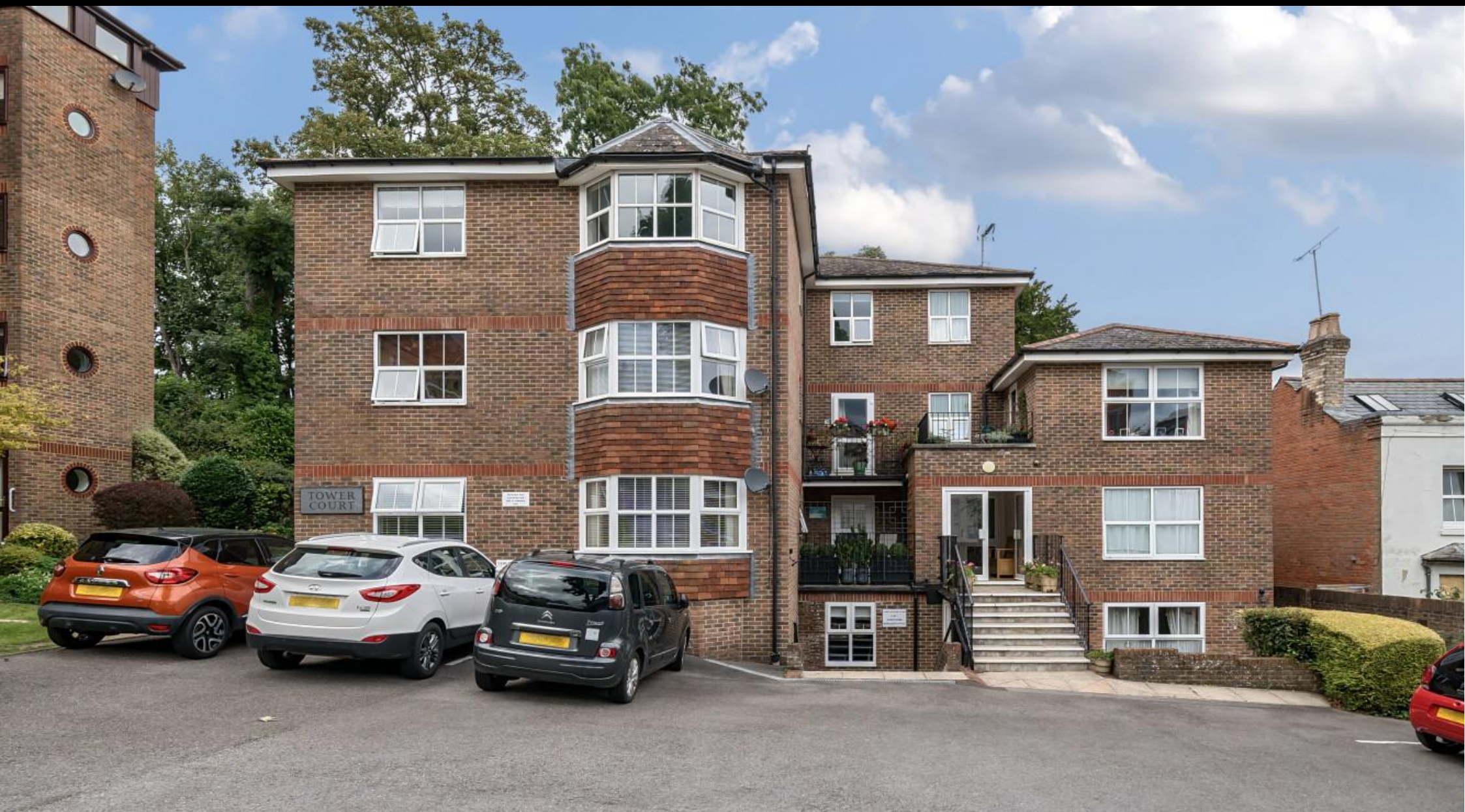
Tower Court, Tower Street, Winchester, Hampshire, SO23 8TA
