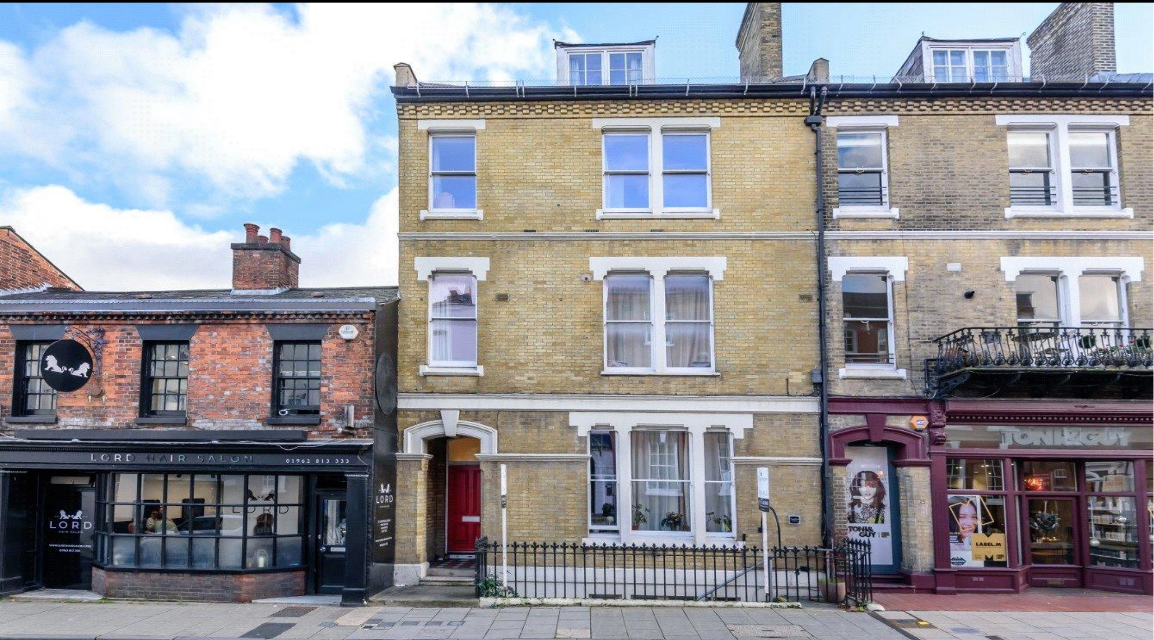
Southgate Street, Winchester, Hampshire, SO23 9DZ
