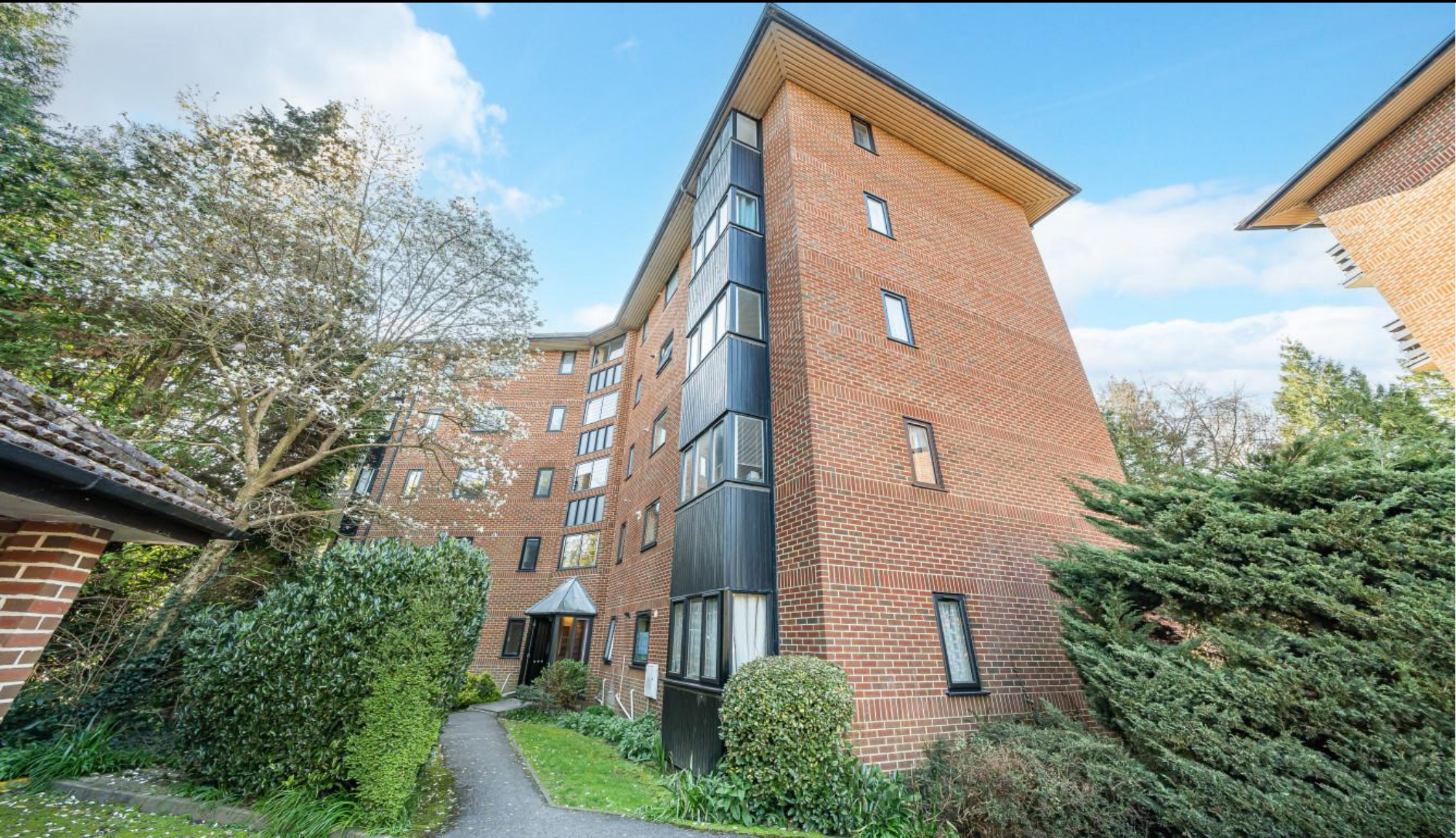
Chelwood Gate, Glen Eyre Road, Bassett, Southampton, Hampshire, SO16 3TZ
