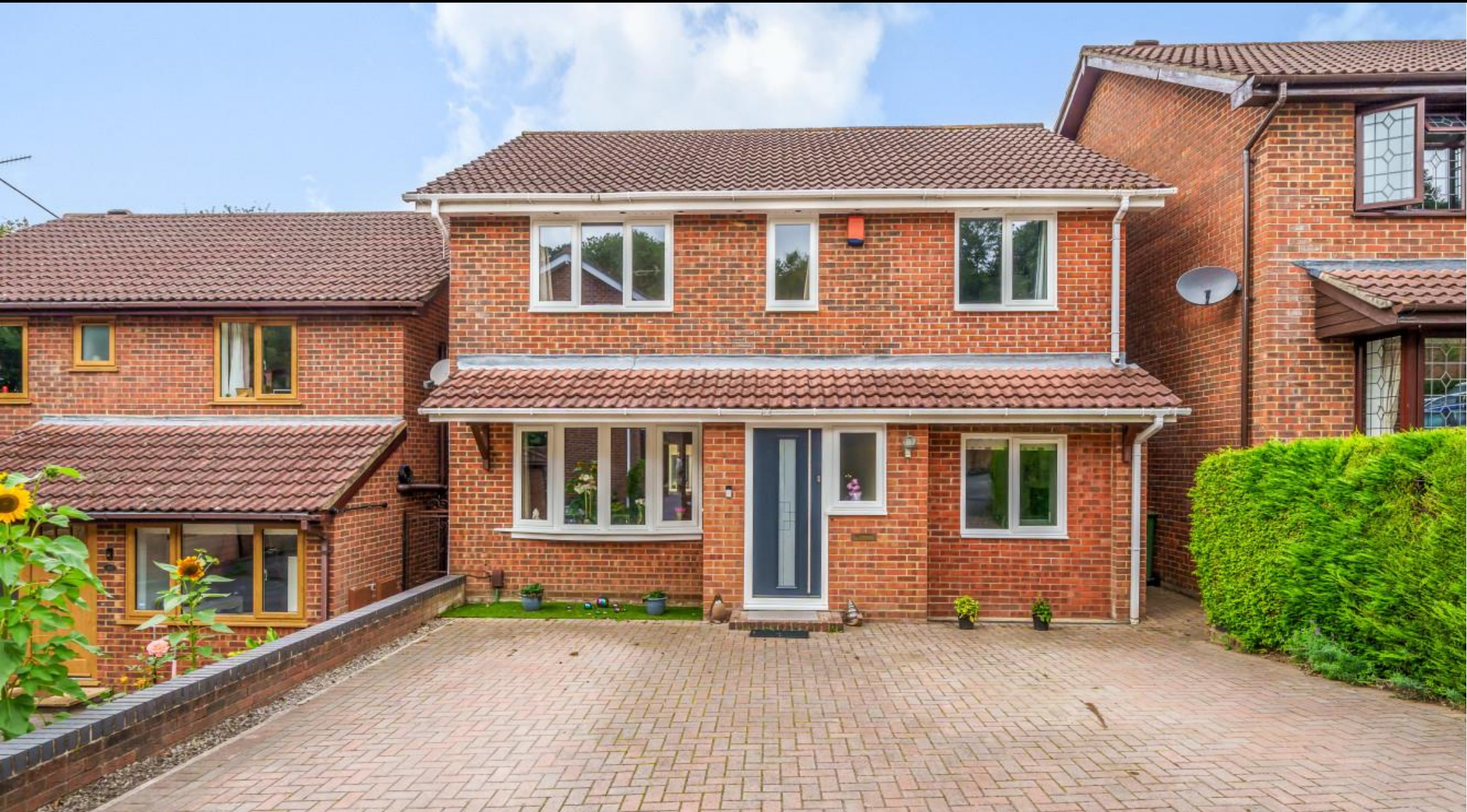
Swincombe Rise, West End, Southampton, Hampshire, SO18 3NL
