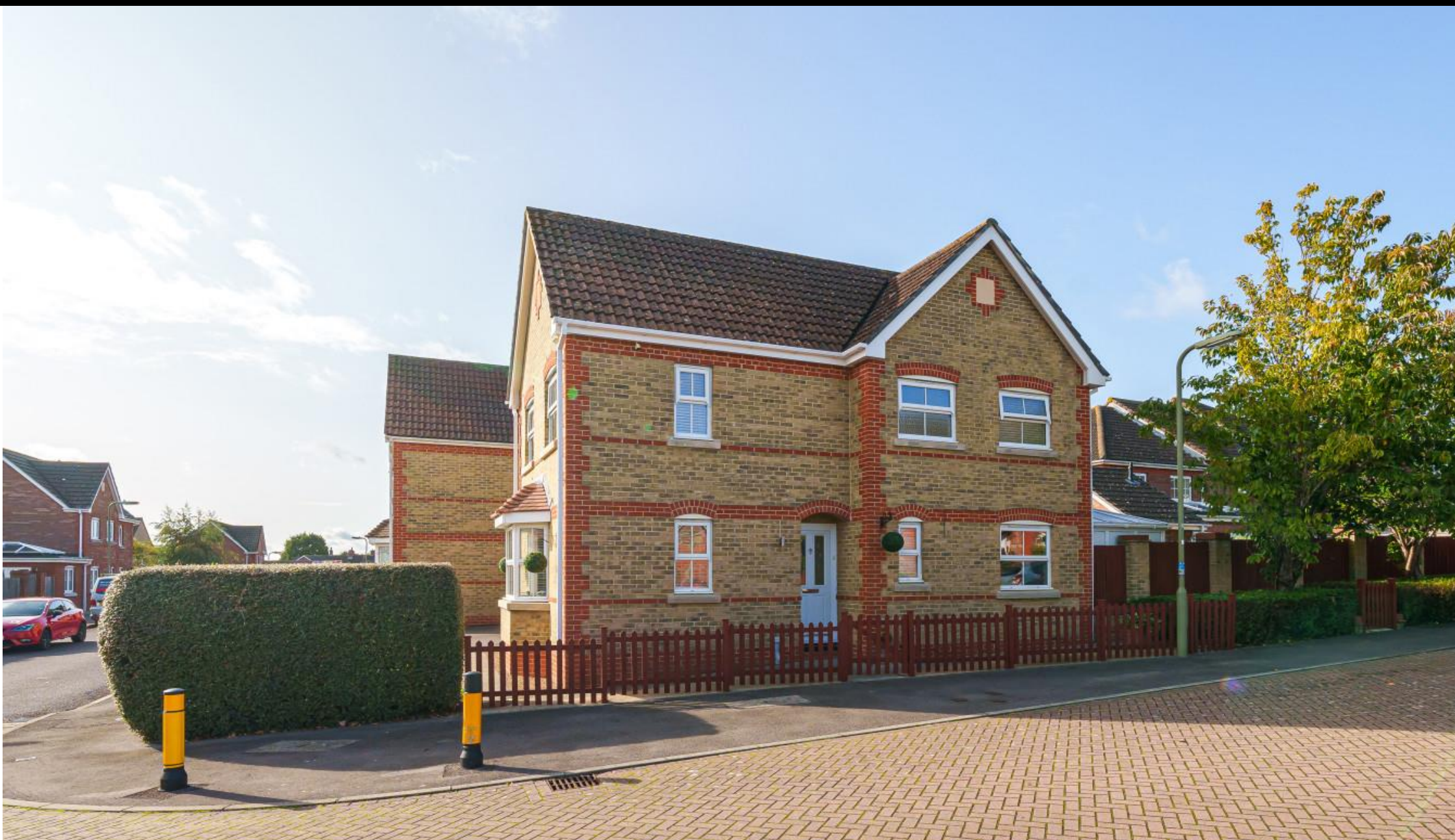
Gardenia Drive, Titchfield Park, Hampshire, PO15 5DN
