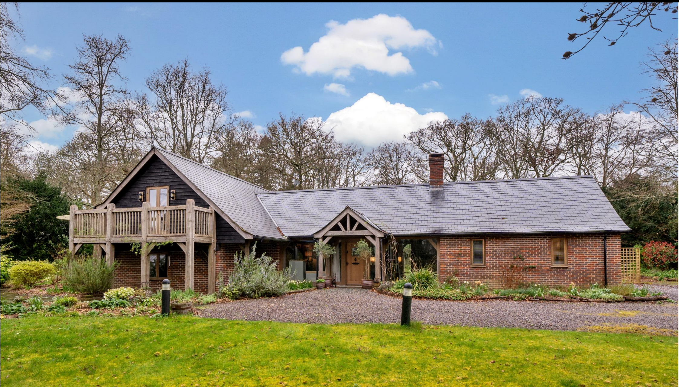
Embley Lane, East Wellow, Romsey, Hampshire, SO51 6DN
