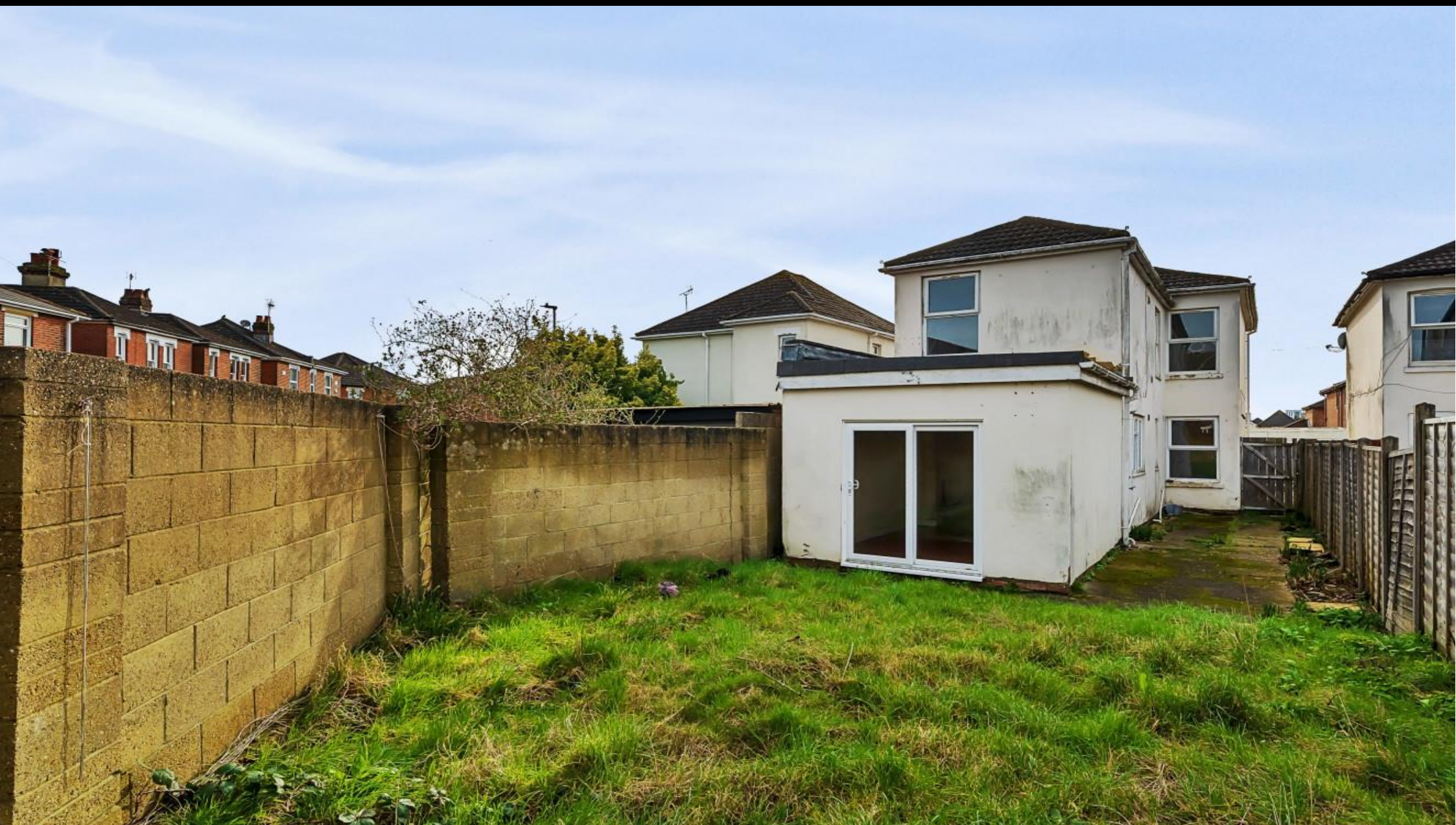
Whitworth Road, Bitterne Park, Southampton, Hampshire, SO18 1GF
