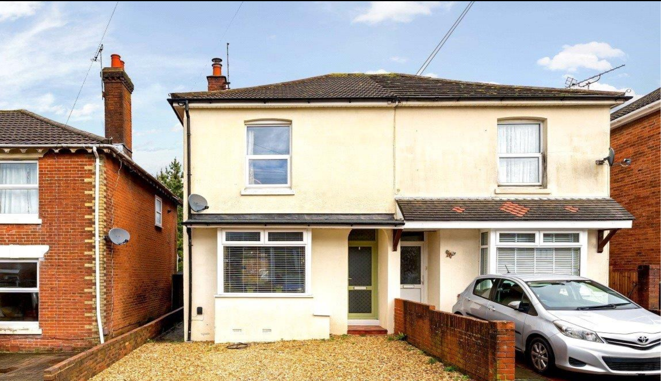
Florence Road, Woolston, Southampton, Hampshire, SO19 9BT
