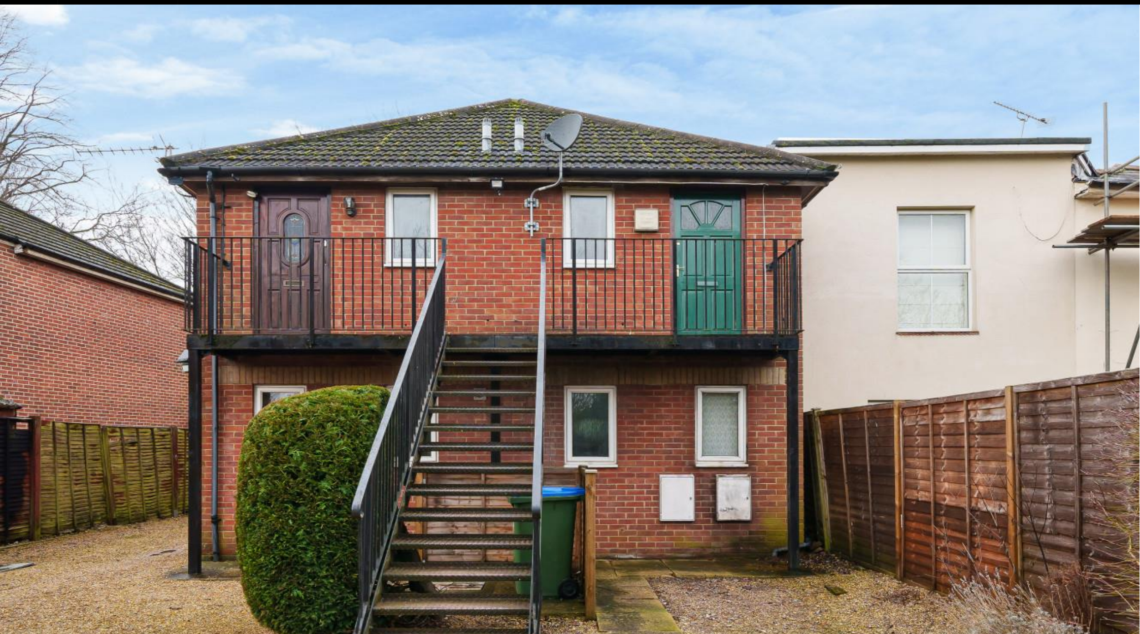
Portswood Road, Portswood, Southampton, Hampshire, SO17 2TD
