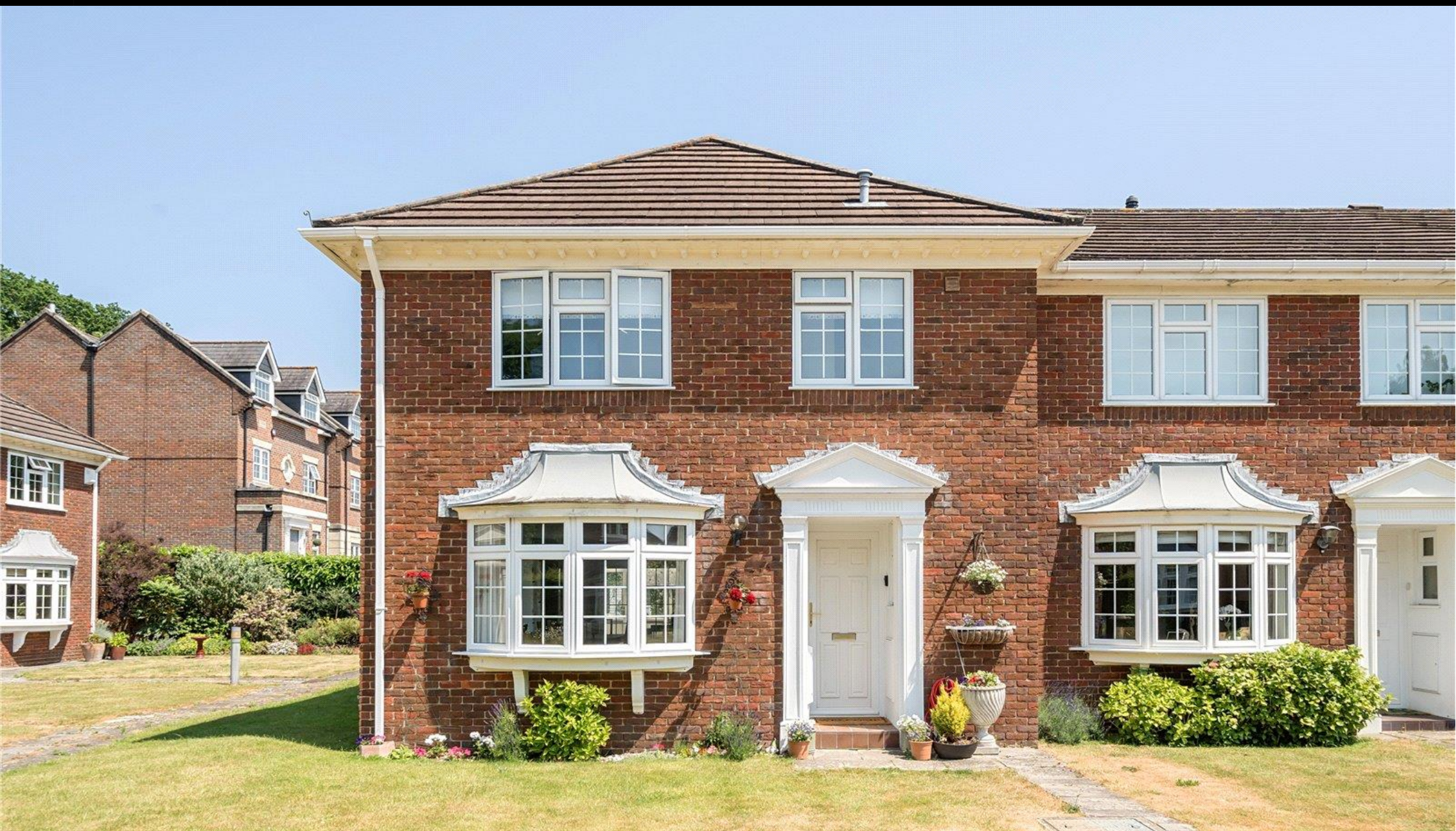
Ashridge Close, Banister Park, Southampton, Hampshire, SO15 2GX
