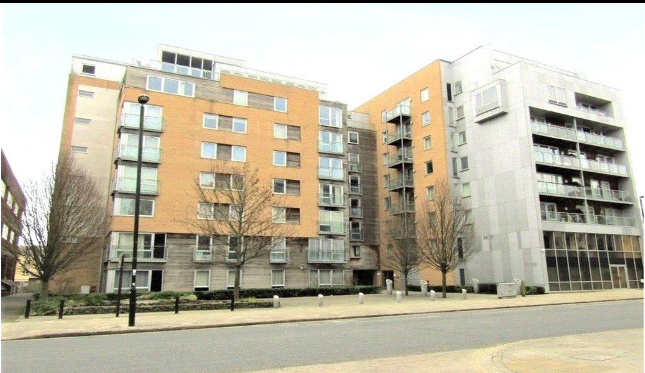
Telephone House, High Street, Southampton, Hampshire, SO14 2NW
