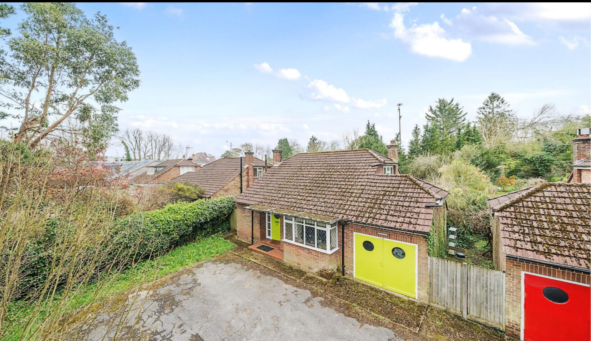
Long Close, Lower Stanmore Lane, Winchester, Hampshire, SO23 9QZ
