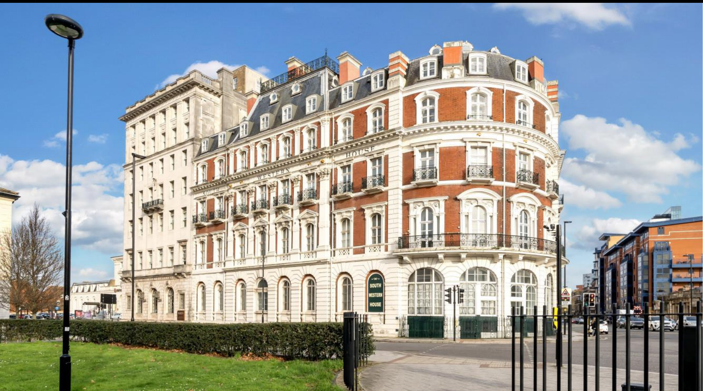
Imperial Apartments, South Western House, Southampton, Hampshire, SO14 3AL
