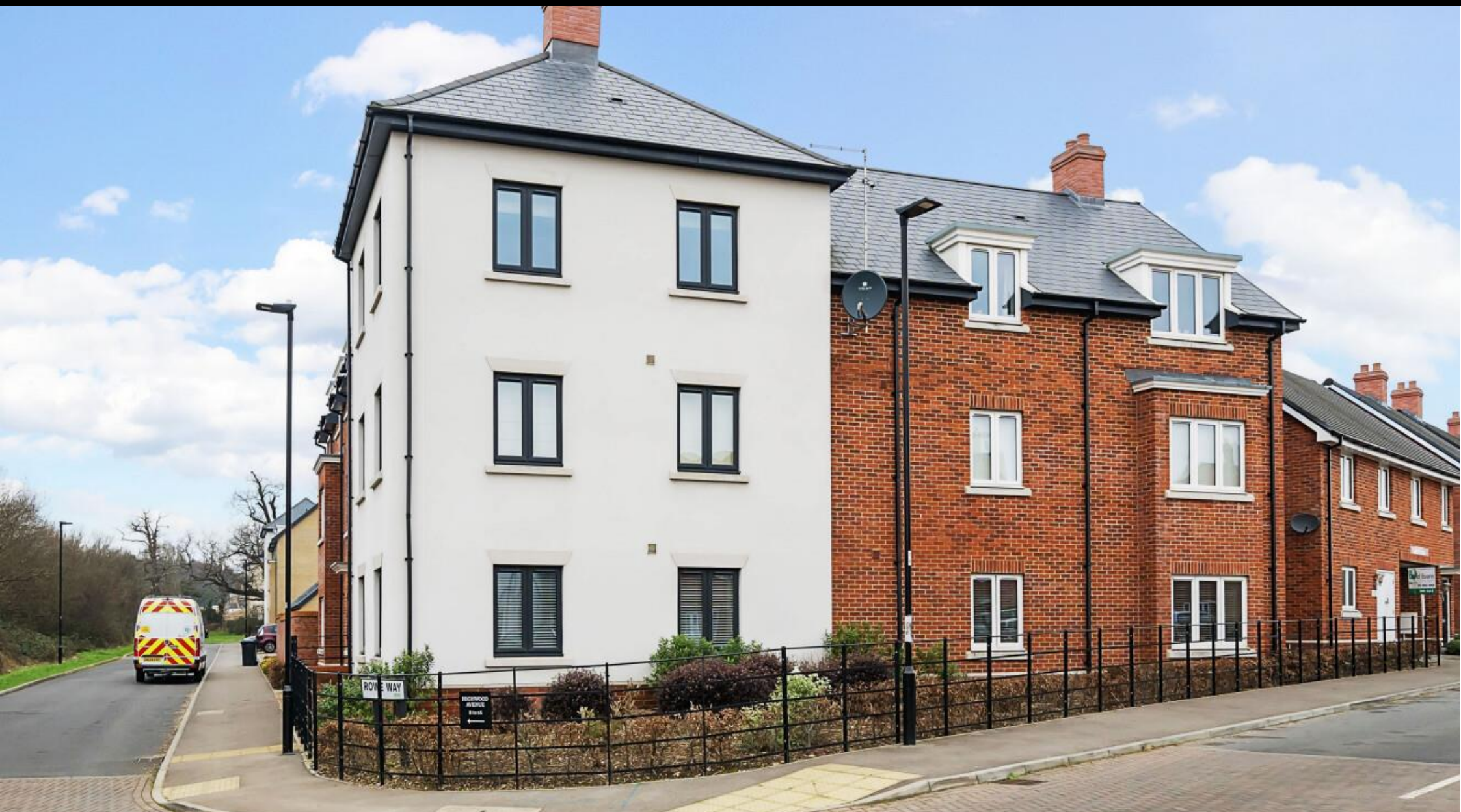
Highwood Avenue, Eastleigh, Hampshire, SO50 9QY
