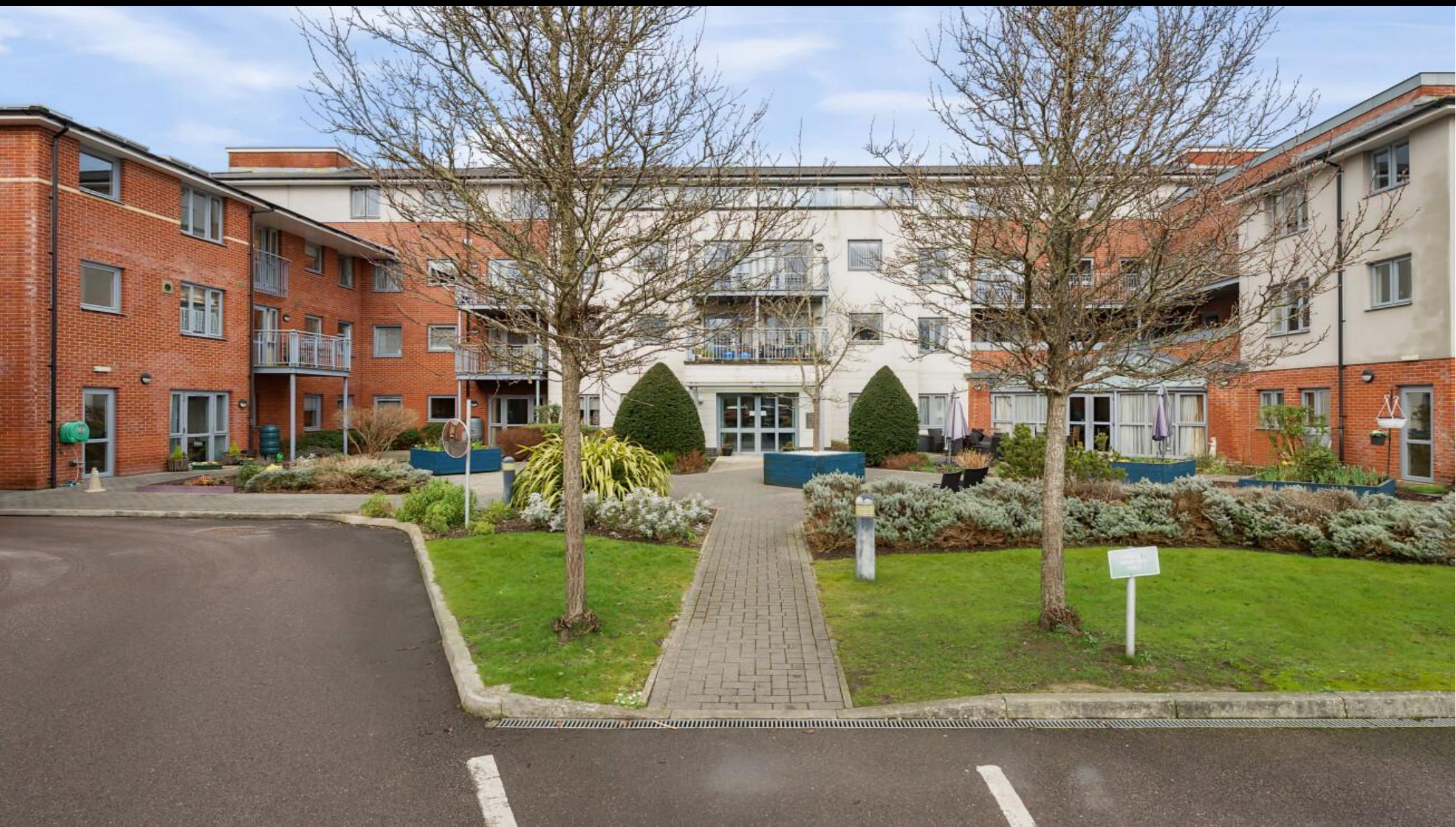
Catherine Court, Sopwith Road, Hampshire, SO50 5LN
