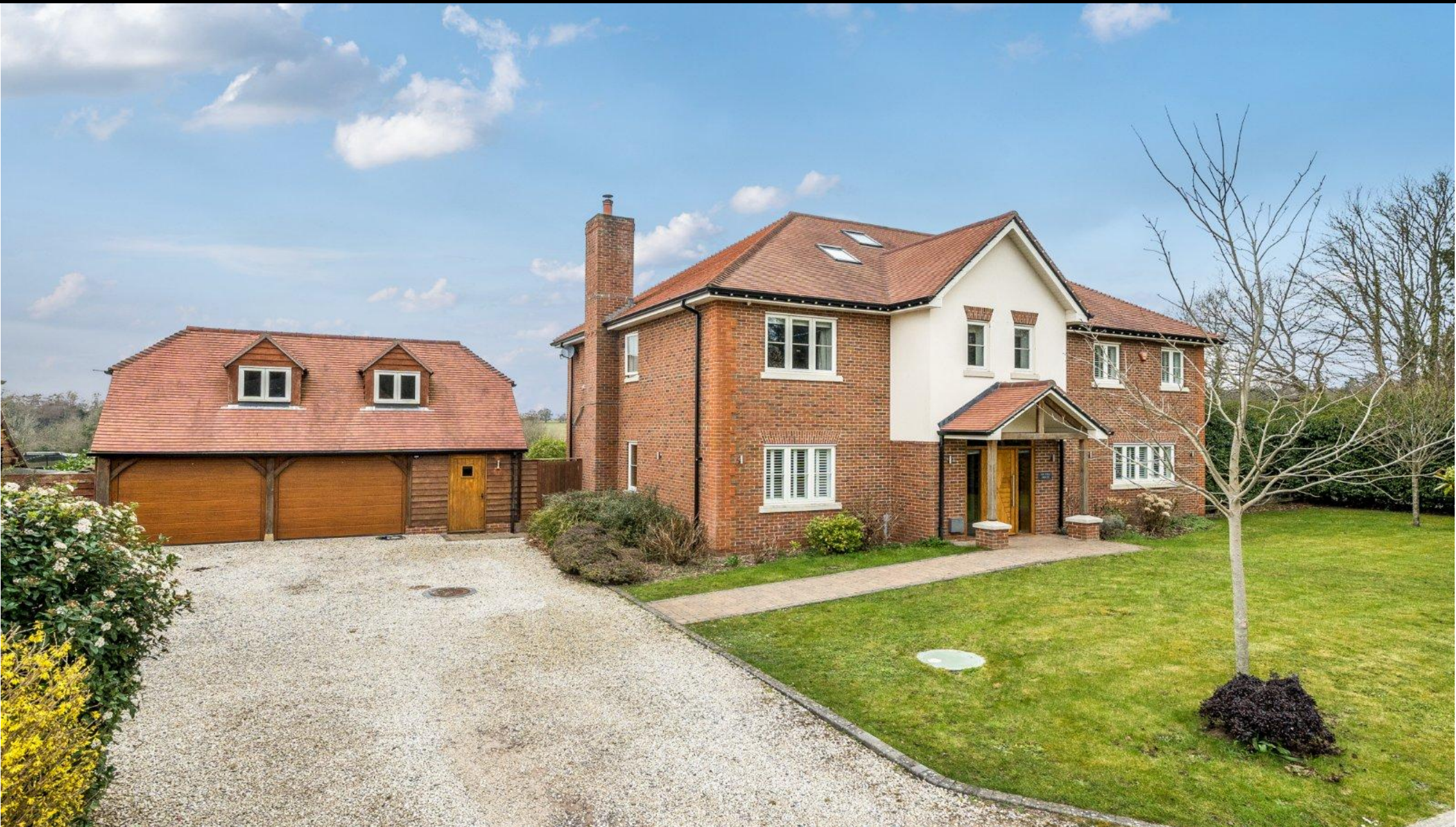
Broadgate Farm, Hook Road, Ampfield, Romsey, SO51 9AU
